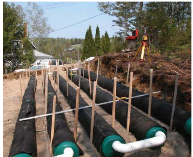
Enviro-Septic® on sloping terrain
